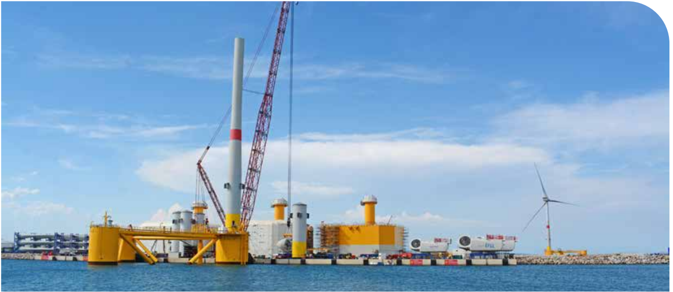
Assembly of wind turbines in Port-la-Nouvelle
